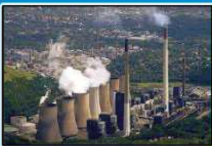
BGR ENERGY (NTTPS STAGE V)
