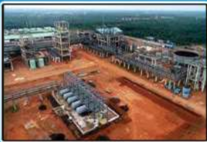
GRASIM INDUSTRIES ELECTRIAL E&C PROJECT
