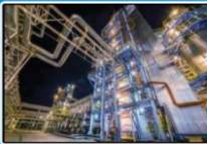
HPCL VIZAG AMC & SHUTDOWN
